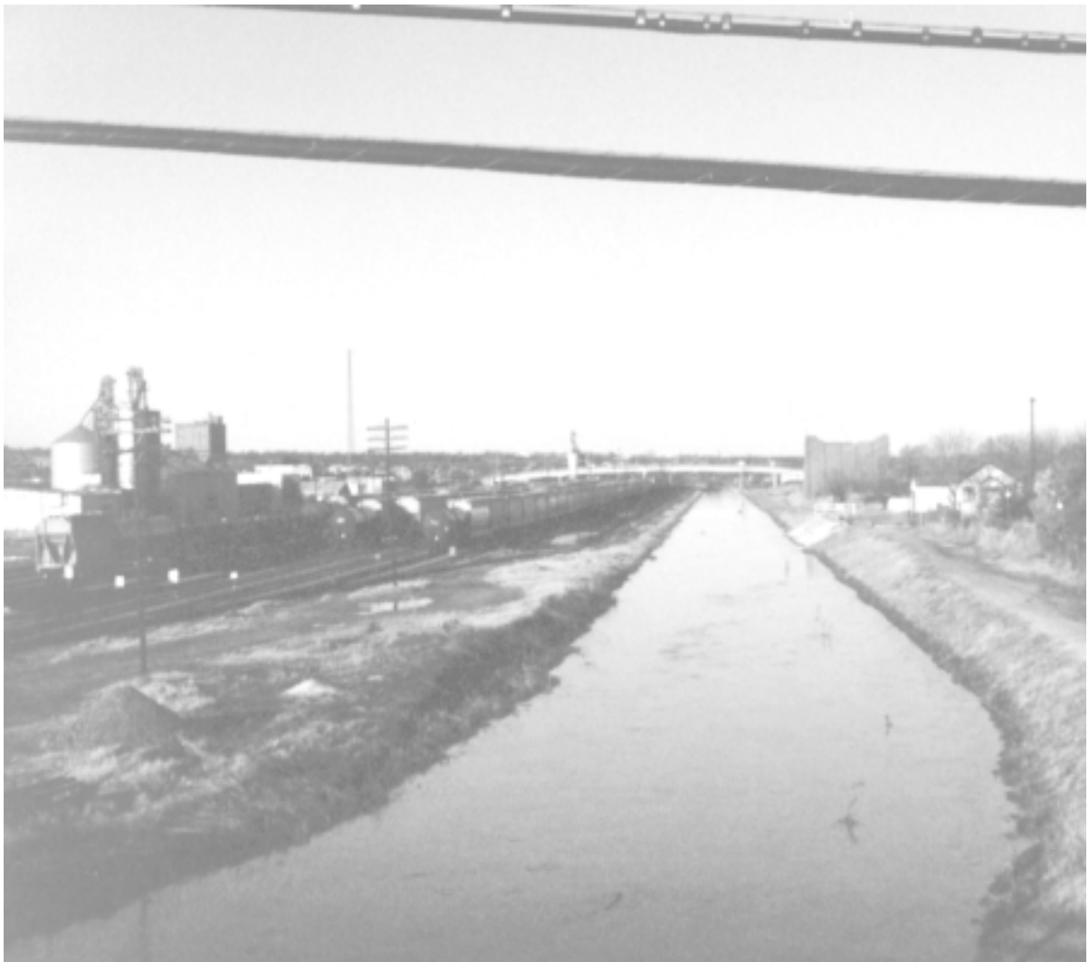
After heavy rains the “ditch” overflows the rail yard.
